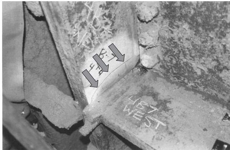
Fig. 1. Divot type connection crack in large section with no gross plastic deformation.
